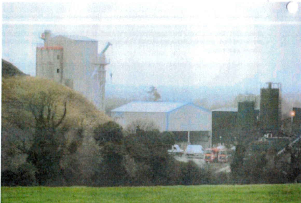
Construction of plant in 2016 without planning consent
